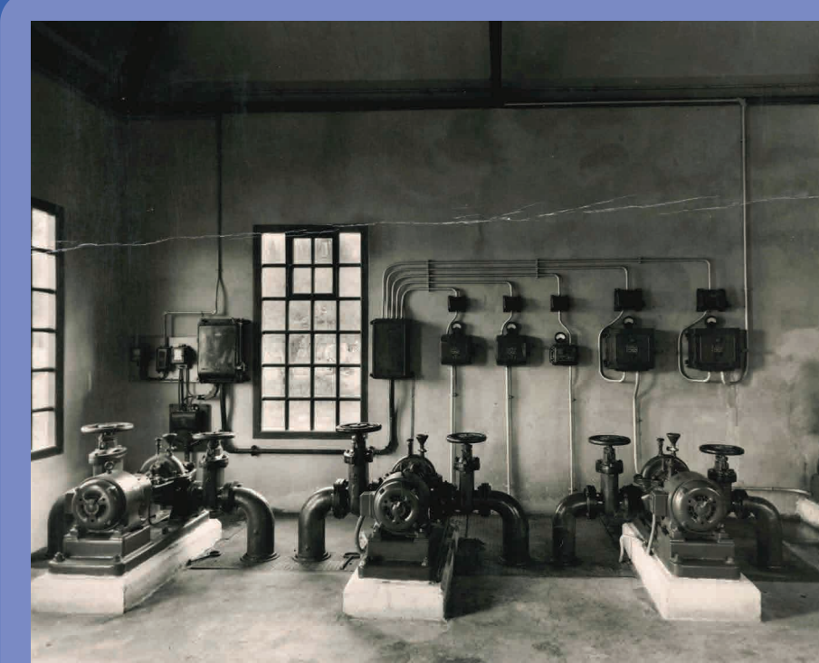
The pumps installed during the 1950's
